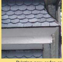
Painting new cedar or pine shake? For long-lasting results dip the shakes in paint prior to installation (coating both sides have proved to give extra life to shakes). Set up a drip collection system so there is less waste, as the paint drips off. Use a paintbrush about 15 minutes after you dip to brush away drips and runs on the end of the shakes.
